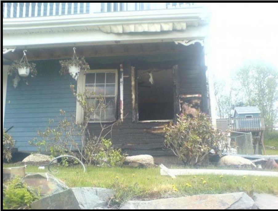
Home burned because of Bark mulch in flower beds, Which caught siding on fire.
