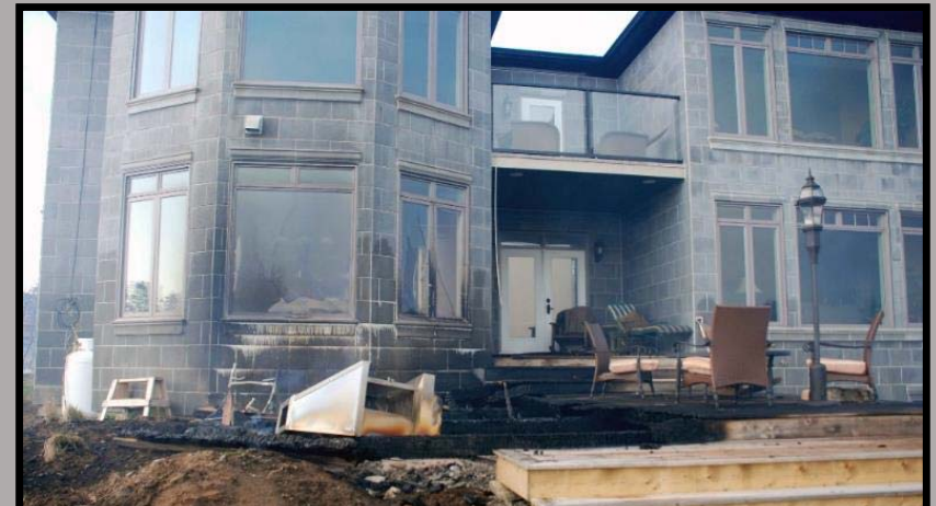
Home survived because of building material – decking may not of burned if lawn furniture was put away
