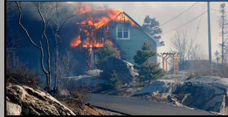
Home burned because of Fire Embers in gutter
